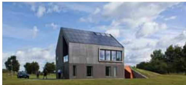
Energy Flex House, Taastrup Henning Larsen
